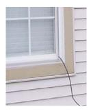
All cable(s) must be routed through the window and/or sliding glass door frame/opening. Penetrating any other surface or material (i.e. bricks, siding, wood, etc.) or running cable(s) outside of the specified area is prohibited as this would involve use of a General Common Element.
